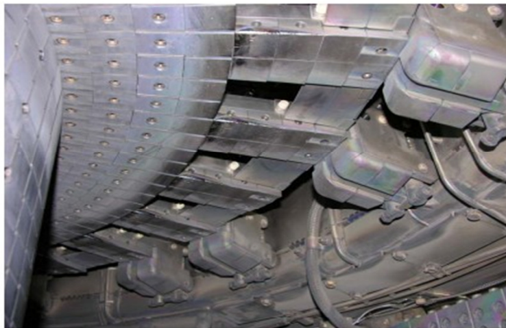
Melt damage at upper edges
